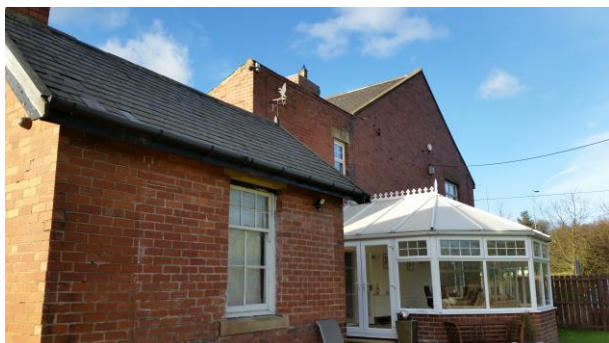
North aspect of the house.
