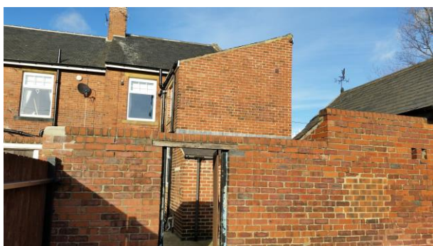
South east aspect of the house showing conservatory on the east side.
